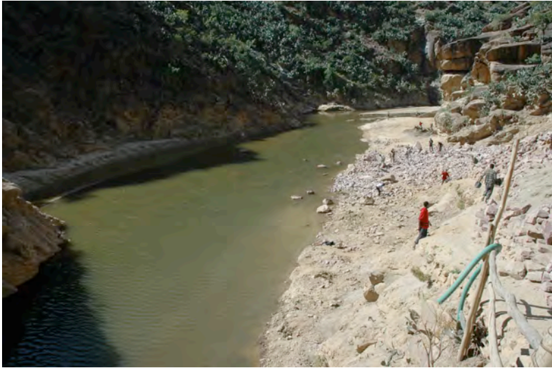
2005, dam body (under construction) at the level of the sluice gate
