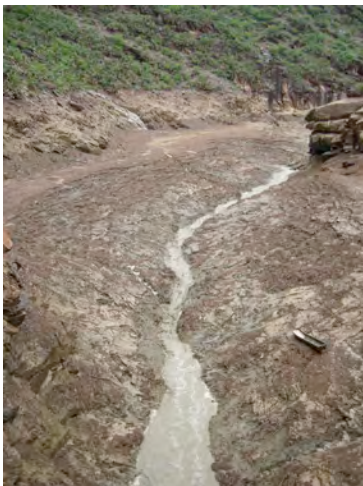
August 2008, shortly before closing of sluice gate
