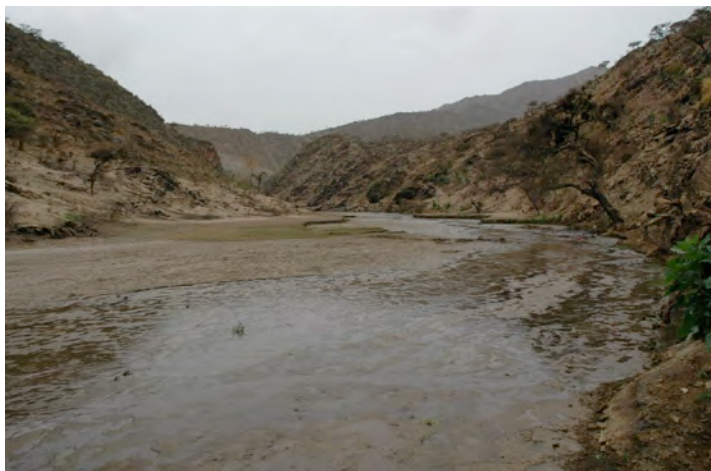
exfiltrating water 800m upstream from dam
